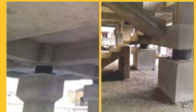
Pictures of Installed Lrb's At Essenza
