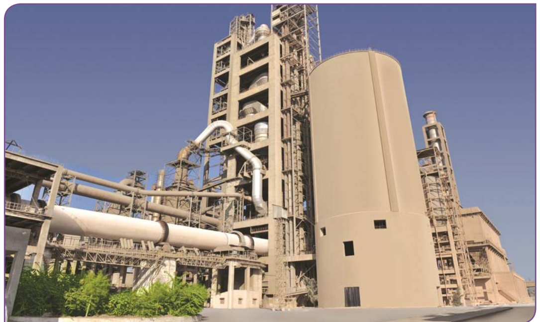
Right: The Sanghi Cement plant in Gujarat was commissioned in 2003. It has an FLSmidth kiln and Loesche mills.
